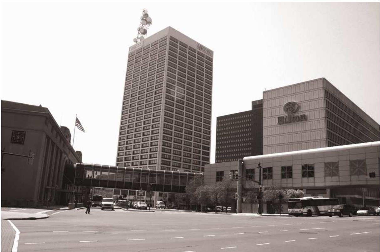
Figure 2 A skywalk connecting Penn Station and the Gateway project (image by NSG).
